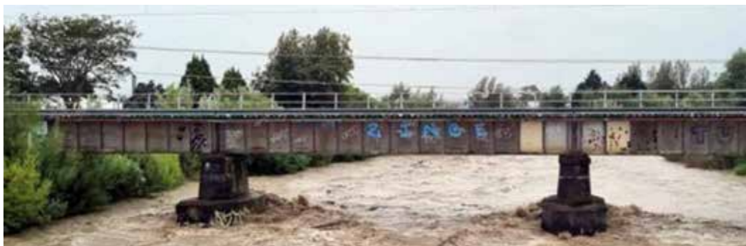
Oroua River runs high at the rail overbridge RNZ Severe weather this summer left tens of thousands of households without power.
