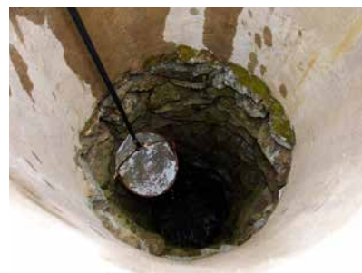
Fresh water is vital to life on land. Over-extraction is dangerous.
